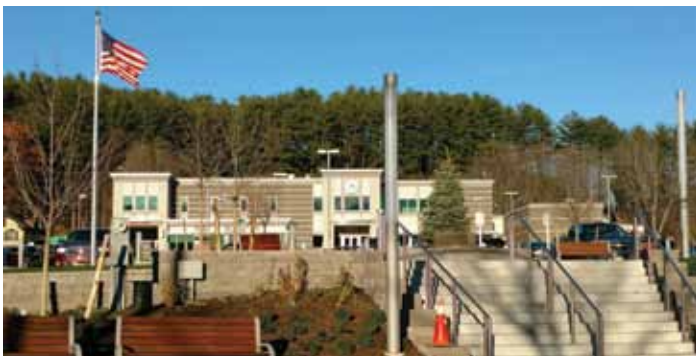
Looking East from Water Street.
